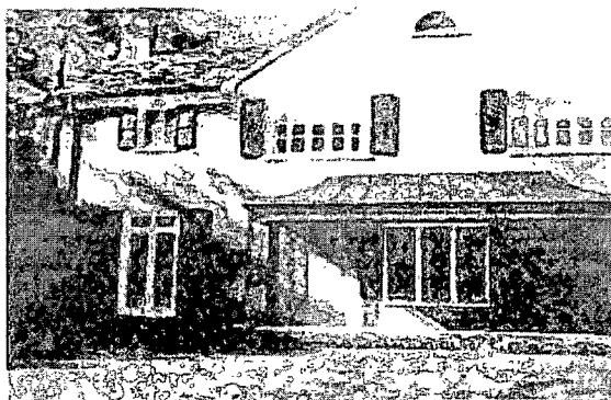
Figure 21-Area overview: North face of home
