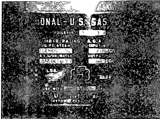
Figure 47-Boiler data plate
