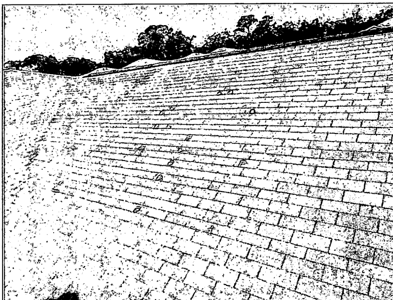
Photograph 24 Randomly selected roof slope. The "B" marks indicate over-driven nails.
