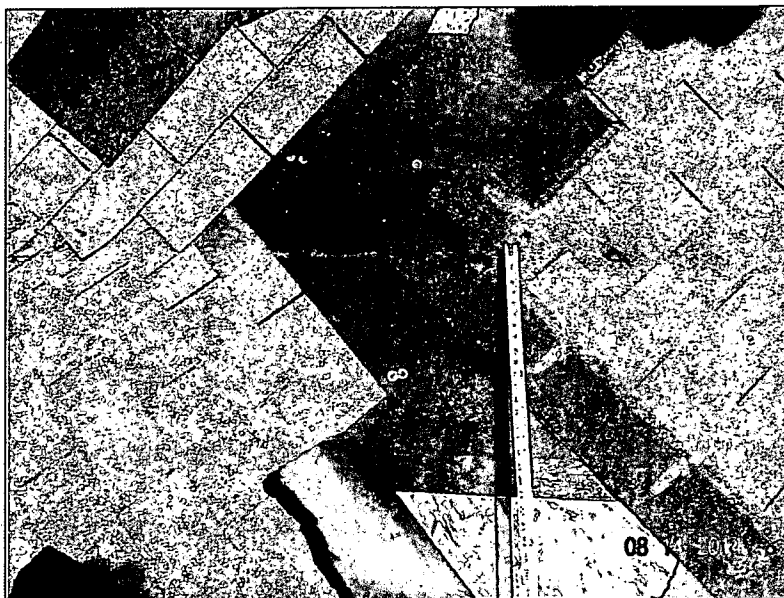
Photograph 24 Randomly selected roof slope. The "B" marks indicate over-driven nails.
