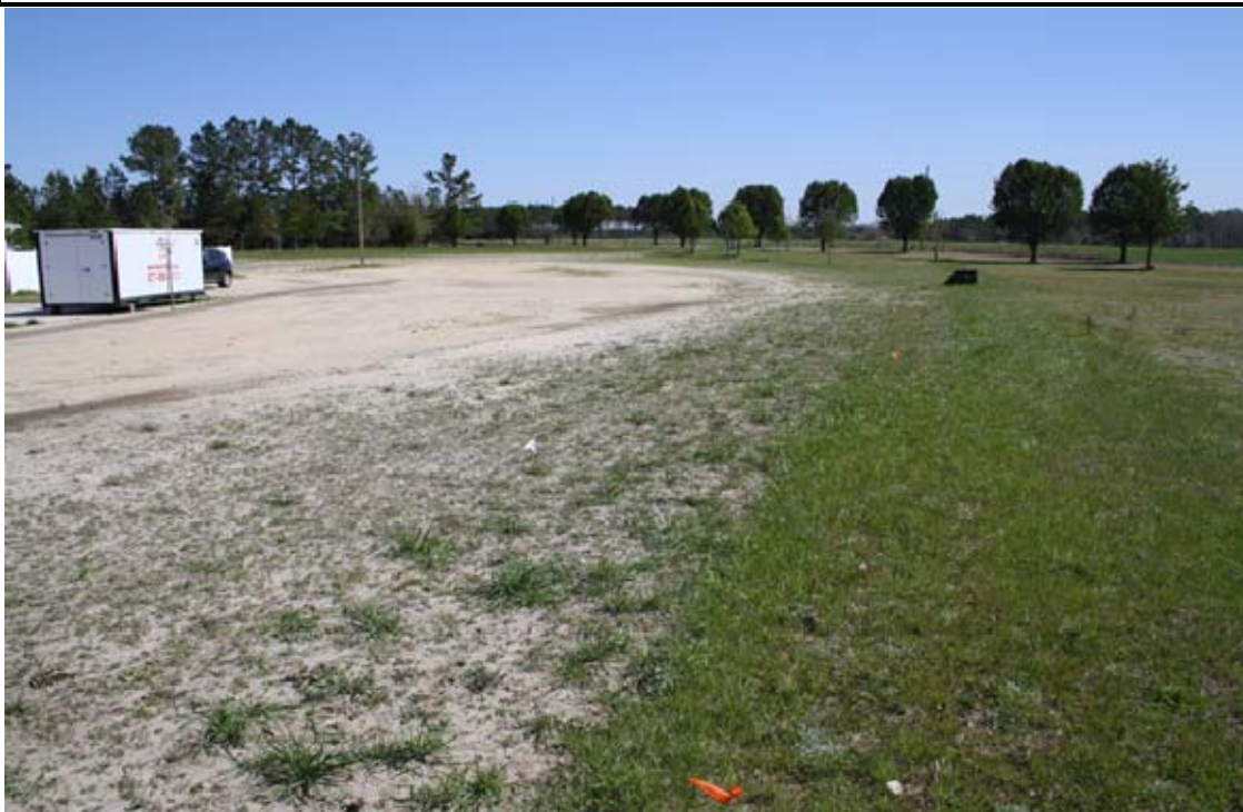
Figure 6. A view along the east side property line showing grading to divert water away from the residence. Note: This work was performed by the homeowner and not the home contractor.
