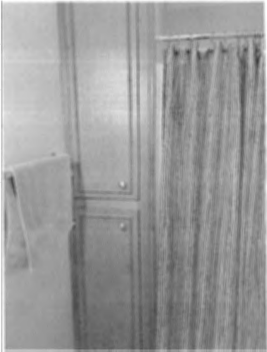
Shower & Linen Closet (Original Pool House Bathroom)
