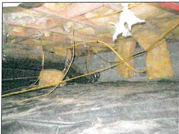
7.5 Item 5(Picture) Hanging insulation
