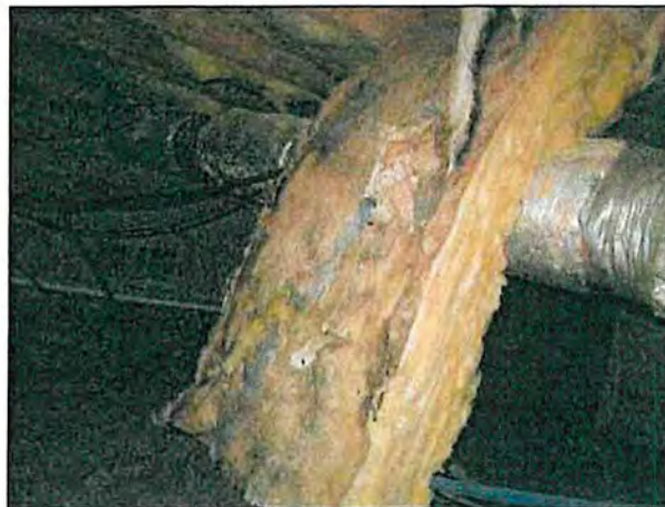
7.5 Item 4(Picture) Hanging insulation
