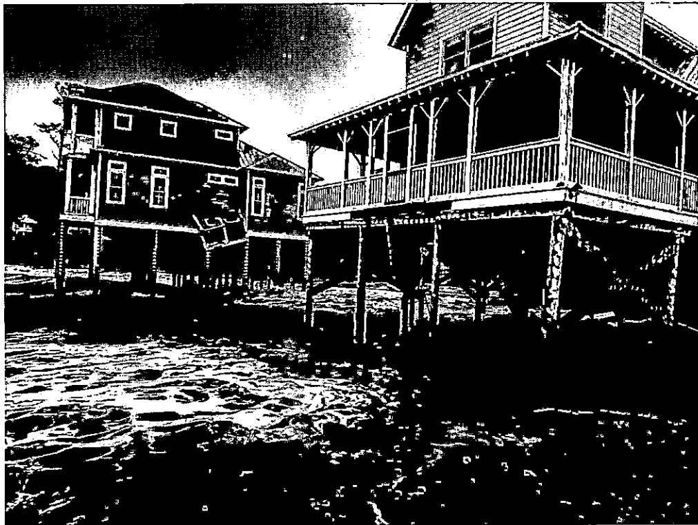
Image 5: Abandoned Properties Immediate South of Noller Residence (formerly 29 and 33 Driftwood Cottage Lane)
