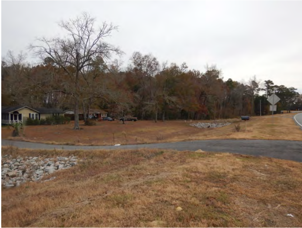
Photo 21 – View of the subject structure and neighboring structure relative to the new road. Photo by ABS taken 12/13/2018.
