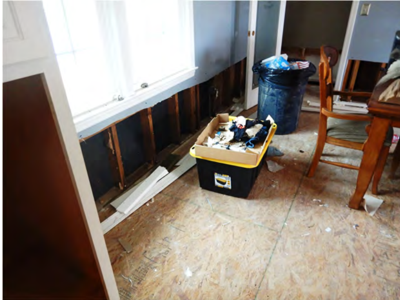
Photo 8 – Interior conditions at the subject structure. Photo by ABS taken 12/13/2018.
