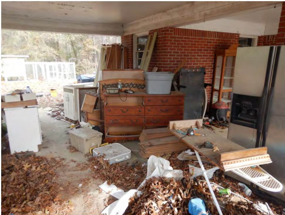
Photo 17 – Damaged contents displaced to the outside. Photo by ABS taken 12/13/2018.
