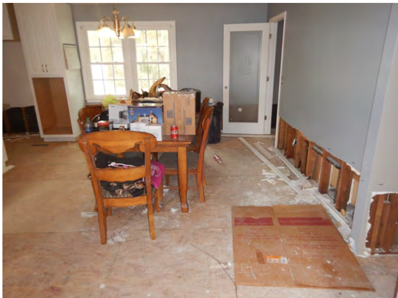
Photo 9 – Interior conditions at the subject structure. Photo by ABS taken 12/13/2018.
