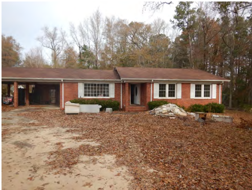
Photo 1 – Partial view of the front (south) elevation of the subject structure. Photo taken by ABS dated 12/13/2018.
