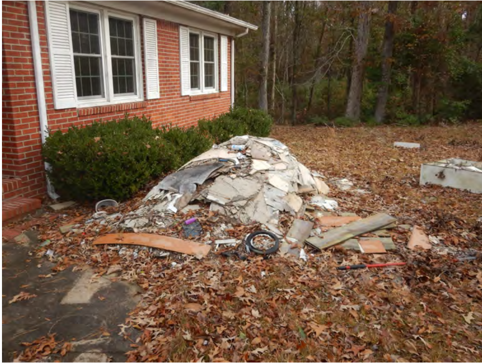
Photo 16 – Flood-damaged interior materials placed in a debris pile outside. Photo by ABS taken 12/13/2018.
