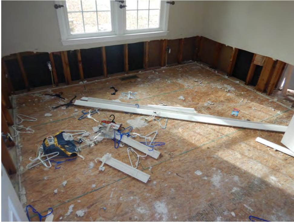
Photo 10 – Interior conditions at the subject structure. Photo by ABS taken 12/13/2018.
