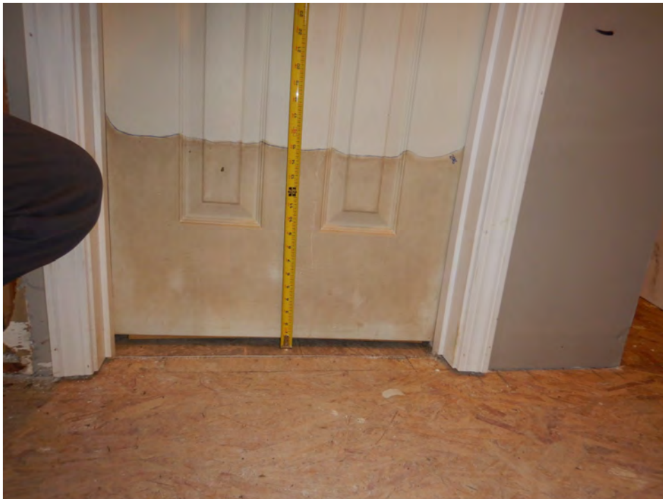
Photo 15 – Interior conditions at the subject structure. Photo by ABS taken 12/13/2018.
