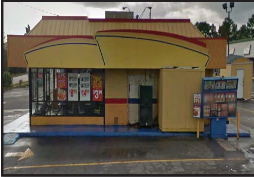
Photo 3: North Elevation & Parking Lot
