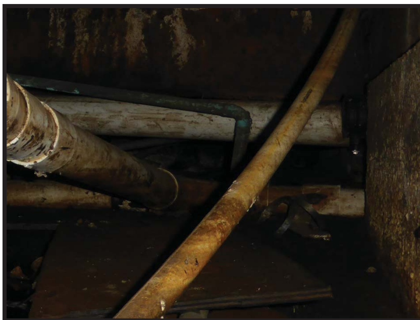
Photo 12: Condition of Under Slab Hung Utilities
