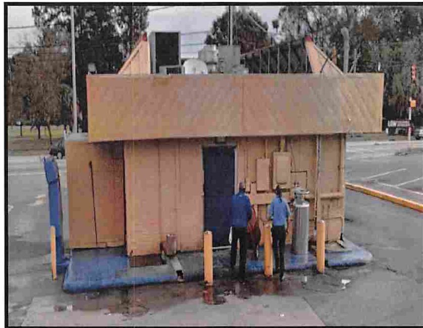
Photo 4: West Elevation & Asphalt Drive-Thru
