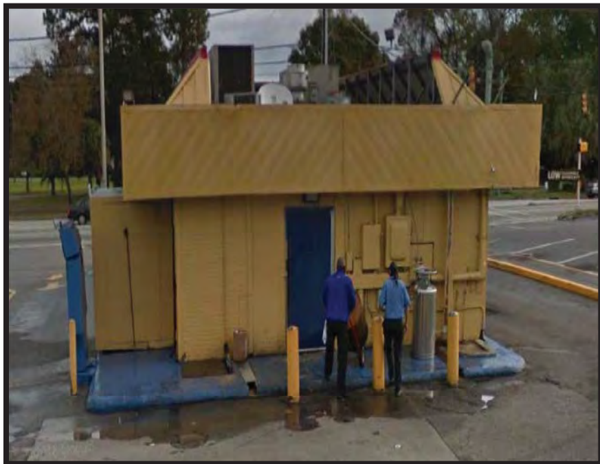
Photo 4: West Elevation & Asphalt Drive-Thru
