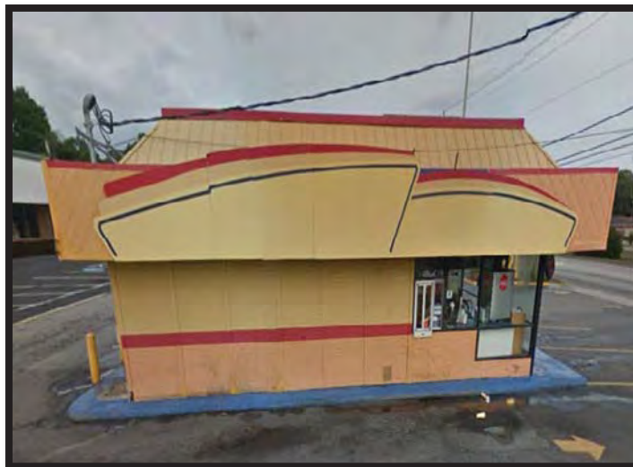
Photo 2: South Elevation & Asphalt Drive-Thru
