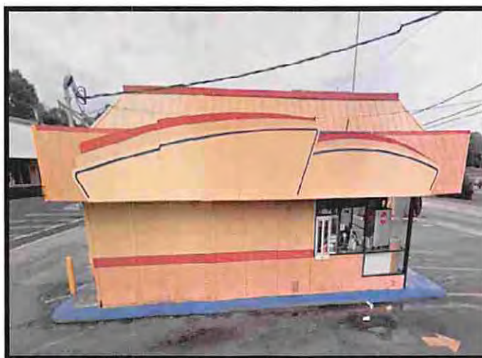
Photo 2: South Elevation & Asphalt Drive-Thru
