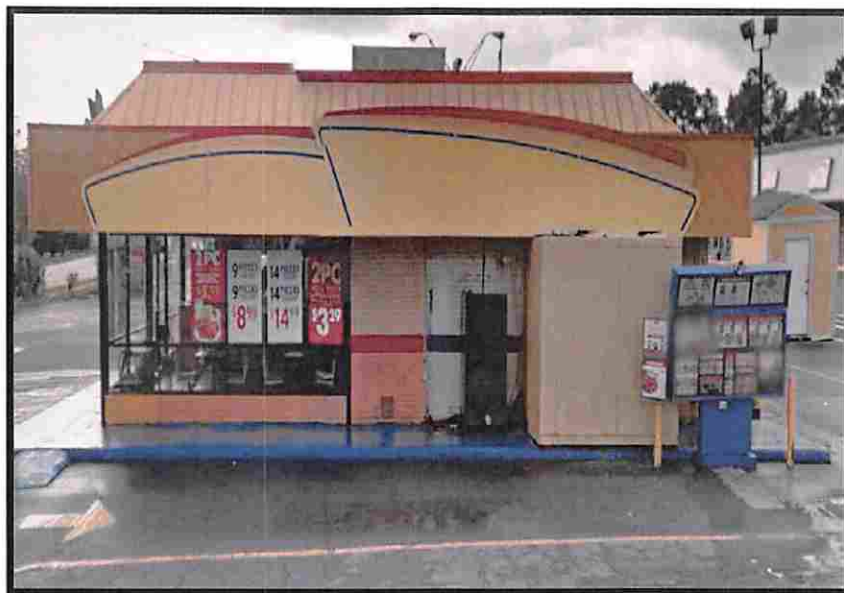
Photo 3: North Elevation & Parking Lot
