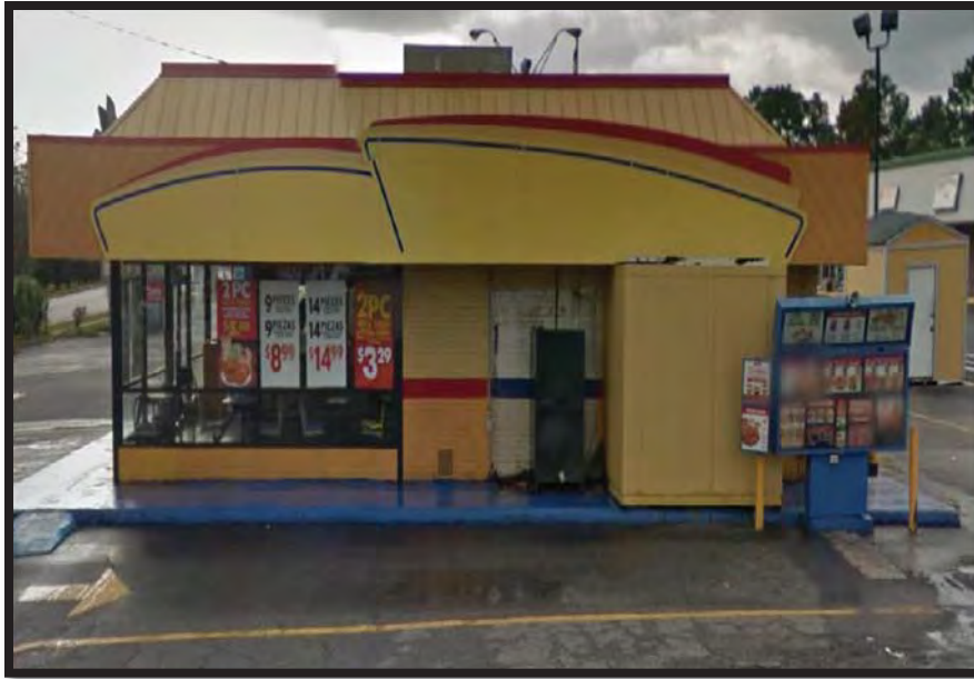
Photo 3: North Elevation & Parking Lot
