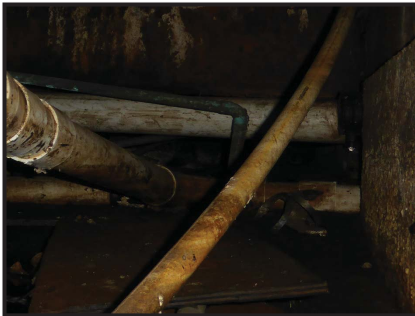
Photo 12: Condition of Under Slab Hung Utilities
