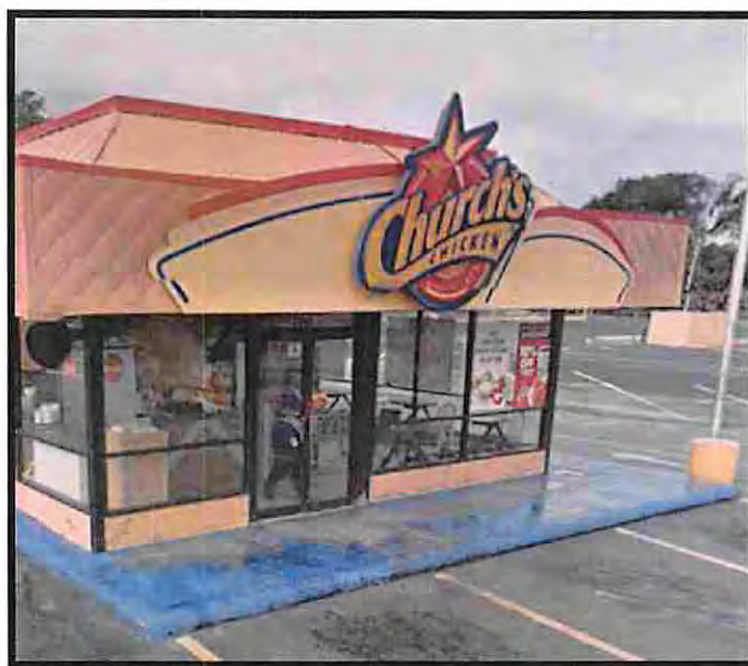
Photo 1: Front/East Elevation & Asphalt Parking
