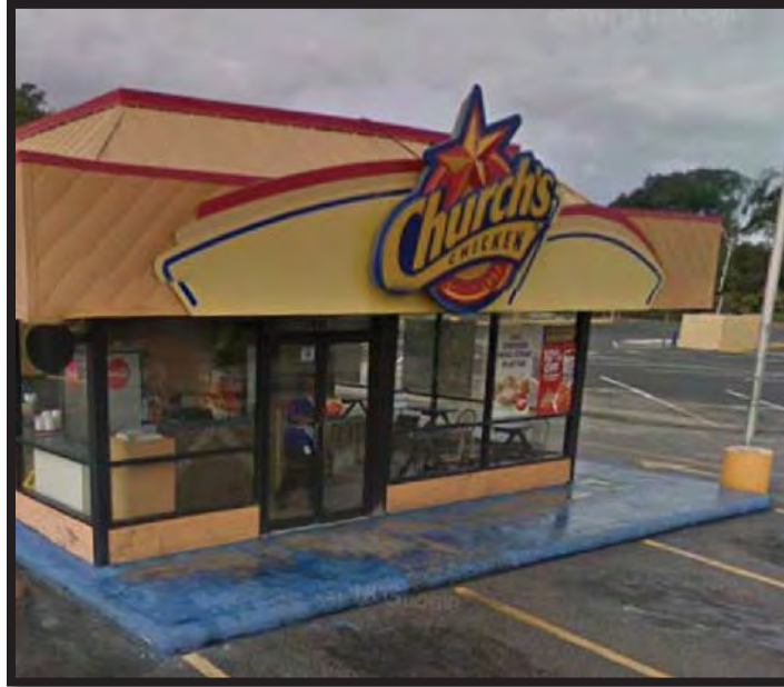
Photo 1: Front/East Elevation & Asphalt Parking
