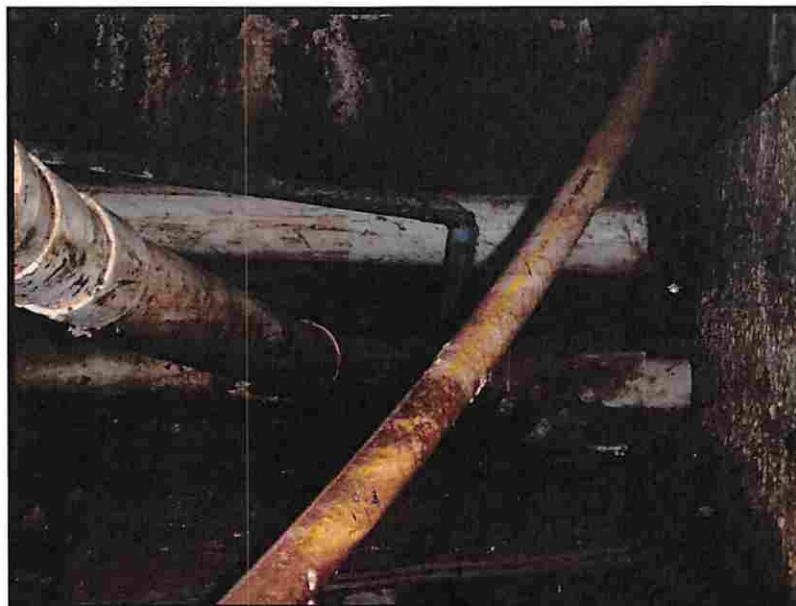
Photo 12: Condition of Under Slab Hung Utilities
