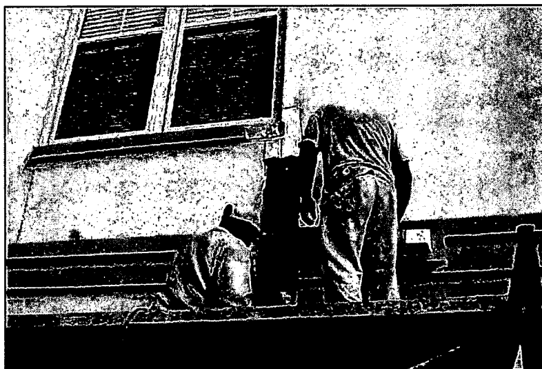
Photograph 6 Note that the deterioration emanated downward from the window, and did not initiate at the decorative band (Photo by WDP).
