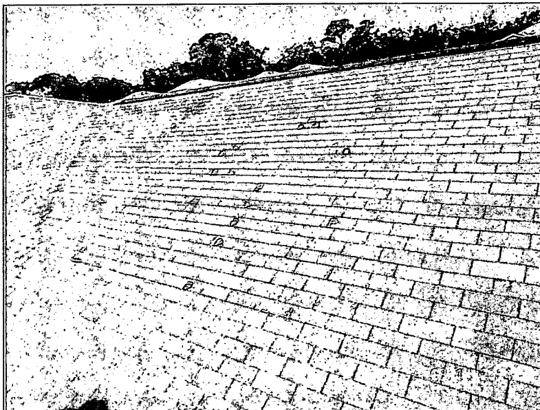
Photograph 24 Randomly selected roof slope. The "B" marks indicate over-driven nails.
