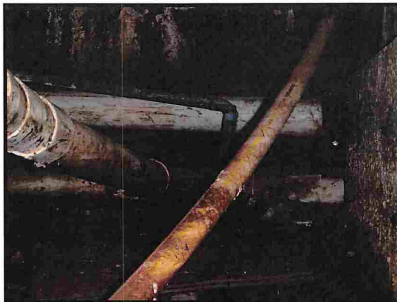
Photo 12: Condition of Under Slab Hung Utilities
