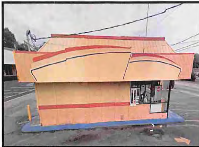
Photo 2: South Elevation & Asphalt Drive-Thru
