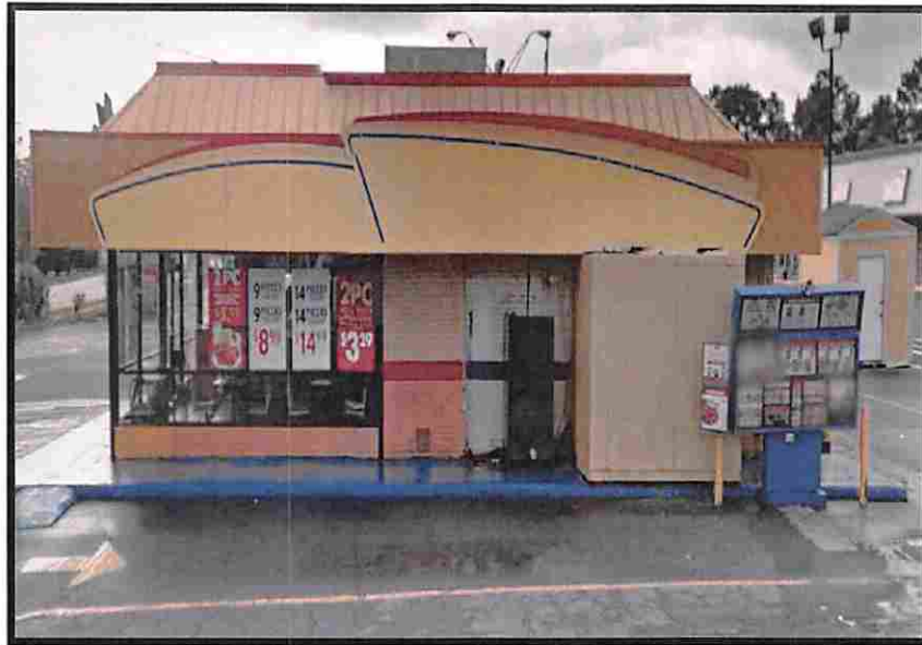
Photo 3: North Elevation & Parking Lot
