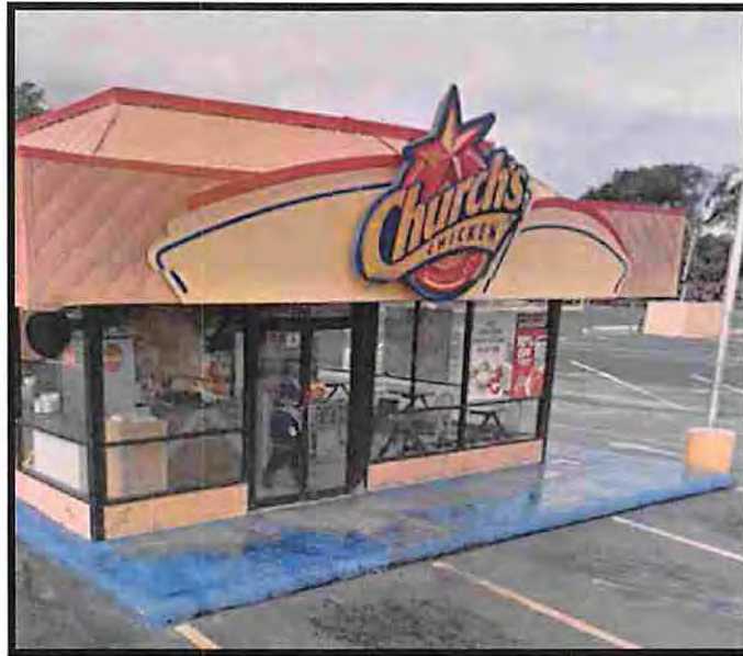
Photo 1: Front/East Elevation & Asphalt Parking
